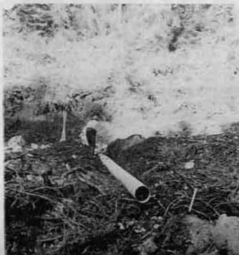
Dynamite can be used for speedy and economical ditching of marshy ground, or . . . below . . . to open the way for laying of a culvert.
