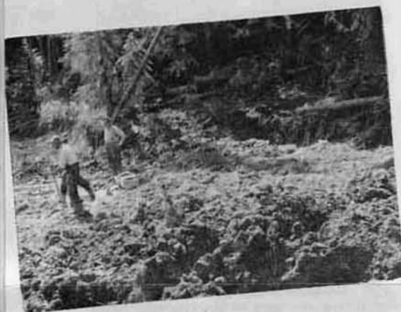
Dynamite can be used for speedy and economical ditching of marshy ground, or . . . below . . . to open the way for laying of a culvert.
