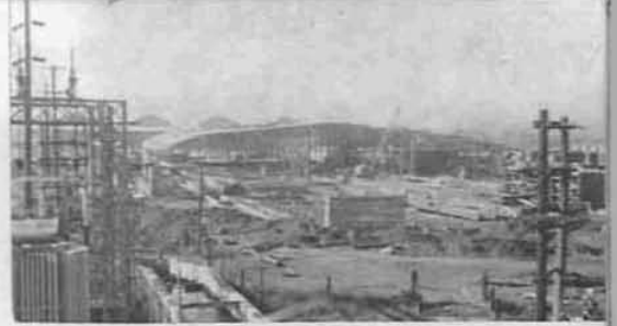
General view of progress of veneer plant.
