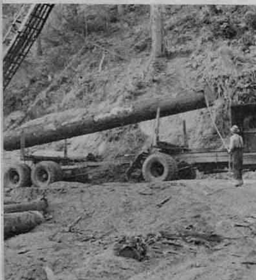
Below . . . truck loading on Bovill side.
