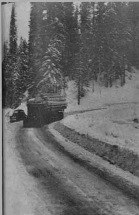
Logging truck riding easily over calcium chloride treated road on Bob's Creek.
