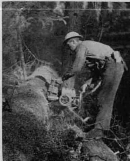
Charles Donahue bucking a log with his one-man chain saw.
