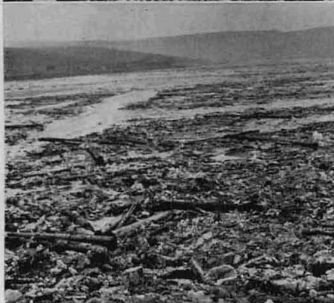
Top scene shows the logs and ice against one of the roller gates at the Clearwater Dam. Lower picture is a view upstream from the mill pond.
