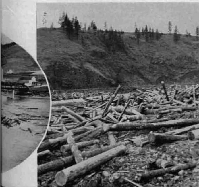
... a jam against the Lenore Bridge. Picture on right shows several
