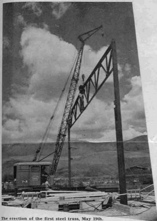
The erection of the first steel truss, May 19th.
