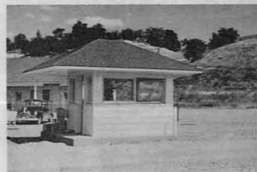
The picture at the top shows an interior view of the time office. In the background Jerry Johnston, pay master, is discussing some business with one of his assistants, Lloyd Southwick. The picture immediately above shows the new gate man's office. Wider driveways for both incoming and outgoing traffic have been provided and the entire entrance takes on a modern and pleasing appearance.
