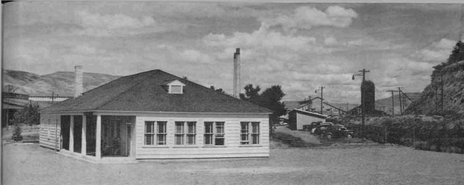
The above view shows the new office which replaced the old time office at the entrance of the Clearwater Unit plant at Lewiston. The new building will house the time office, fuel office, interview office for prospective employees and a visitors assembly point prior to the tour of the plant.
