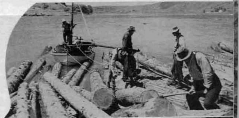
Securing boom from power boat to log jam. Winch mounted on boat pulls logs from jam into water with wire rope.
