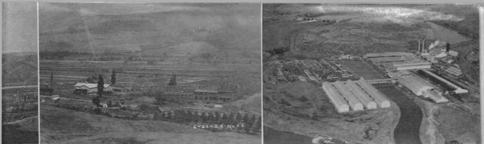
the area in east Lewiston to the modern industrial are now part of the mill pond. Center shows on the left and the frame-work for the sawmill
