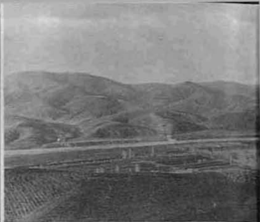
The above pictures show the transformation of a farm into a mill site. Left shows the farms and orchards. Right shows the start of construction with the machinery.
