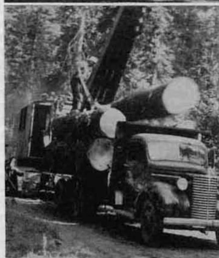
Above: Skidding out a big one at Camp T with a line from a Link Belt shovel. Lower: Loading the same log onto a truck without missing a stroke.
