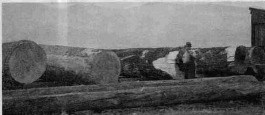
Here are five of the six big logs brought down from Camp T and which had to be hewed off at the swell-ends so they could go through a band saw rig.
