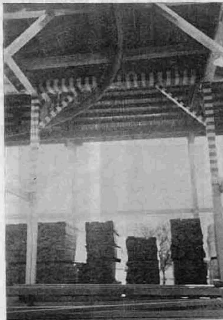
These striped timbers are not related to a zebra. They have been painted orange and black near each switch on the monorail tracks to tell the monorail drivers where the switches are. This is a safety device at the Clearwater unit.
