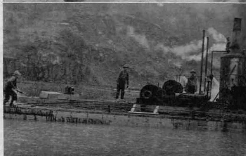
Here is the Potlatch navy. A craft designed for multiple use such as ice-breaker, pile driver, sky-line rig and sea-going donkey engine on the pond, recently took to the water in a formal launching. The upper view shows the barge on the skids; lower, riding at anchor, queen of the waves, and steam up.
