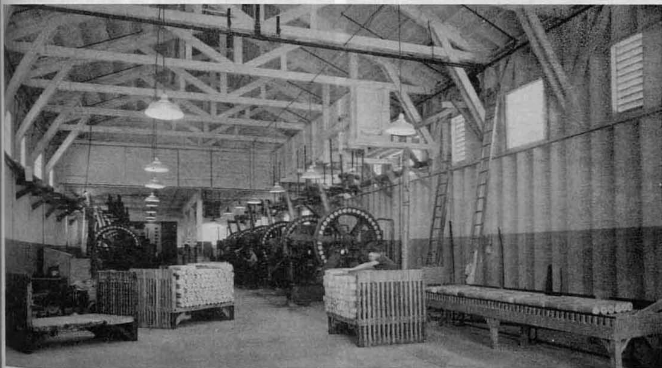
Building an additional 130 feet on the Pres-to-logs plant of the Clearwater unit, the company now has the largest plant of its kind in the world. There are nine machines in operation.
