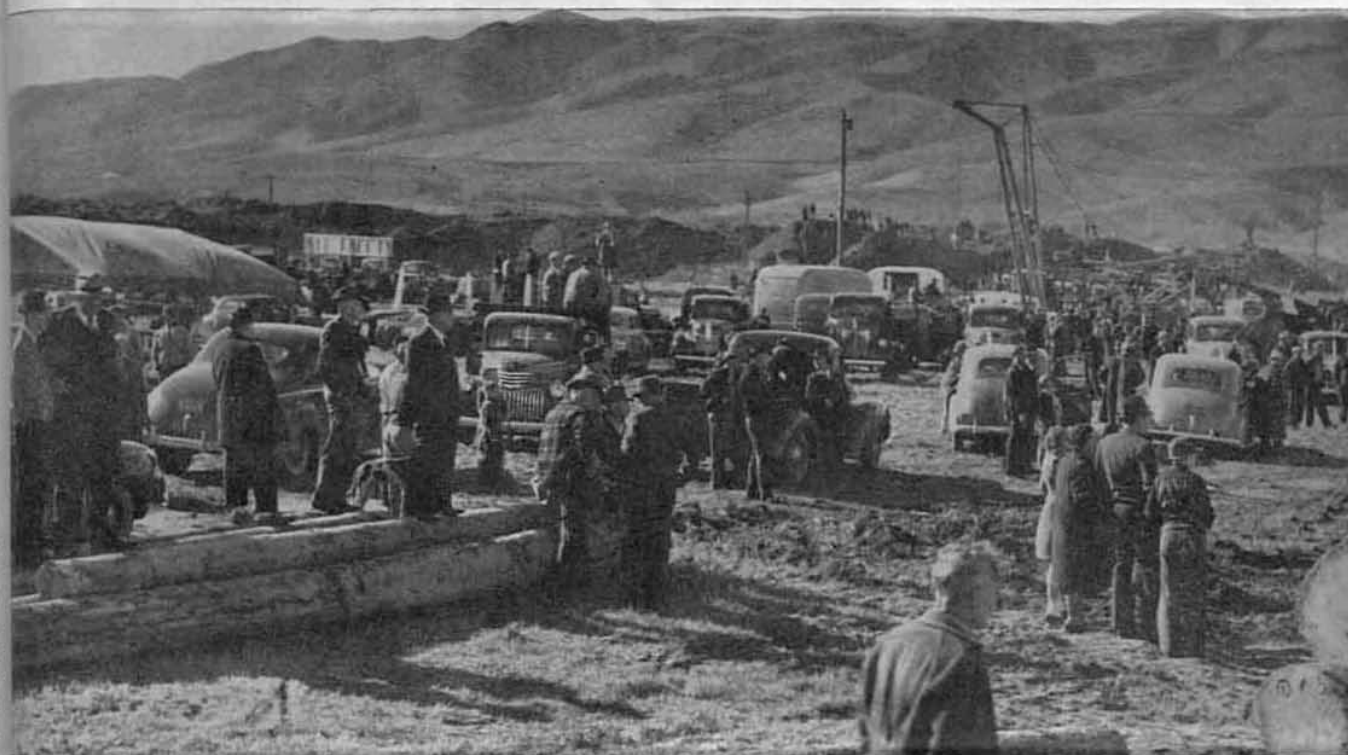
Above: Part of the gallery of watchers at the Intermountain Logging Conference, following a truck load of logs to an improvised landing on grounds of the company's Clearwater unit plant. The Osgood loader's swing boom and engine housing may be seen in the background.
