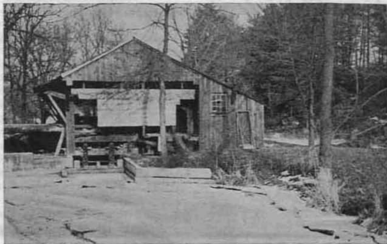
For the past 125 years, this water power mill has been in operation. It is owned by the Rote Brothers, Spring Mills, Pa., and is equipped with a circular saw. Under a good head of water it can cut about 300 board feet per hour.
