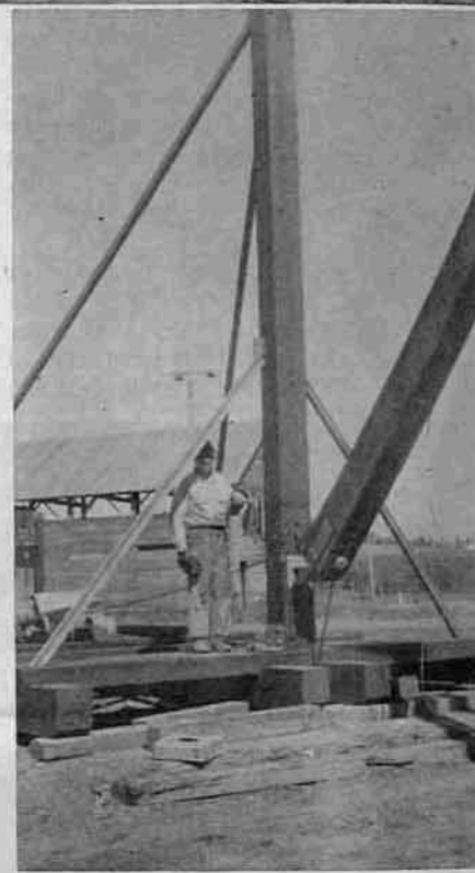
Above is a full view of the new unloader at the Potlatch pond which was designed and constructed by R. E. Owens, foreman of maintenance and construction at that unit. Besides being a time-saver it has a safety factor that keeps truckers out of the path of falling logs, the operation of the unloader being a push button device at a safe distance from the load.
