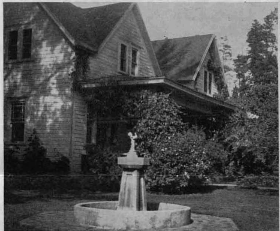
The upper picture shows the old log walls of a cabin believed built in the Potlatch area about 1865, uncovered recently when the sheathing of what was thought to have been just a wooden shack was torn loose. The roof has been removed. The lower scene is that of the W. E. Hearn place on which the old building was situated and revealed when Mr. Hearn decided to do away with the unsightly shack.
