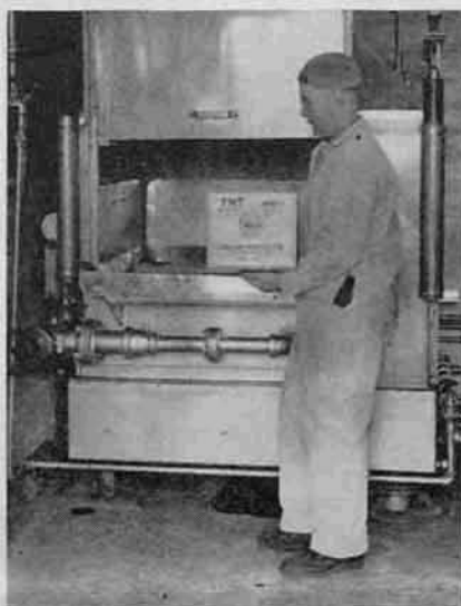
Left: Bulk TNT is being placed in a steam heated melting unit. Right: Liquid TNT being poured into 20-pound aircraft bombs.
