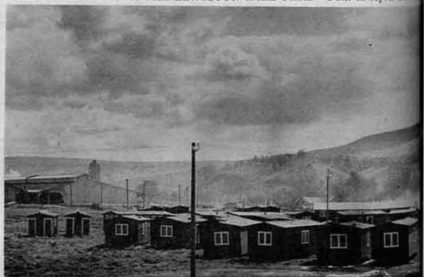
CAMP BUILDINGS IN THE LEWISTON MILL YARD—Built in April and May
