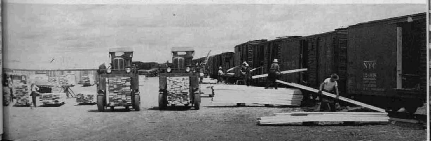
LUMBER CITY—Lumber was the primary building material
