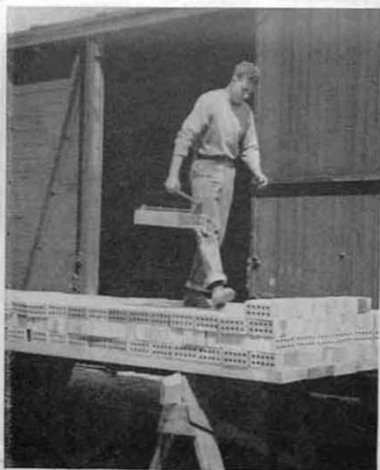
Cored Brick for Rutledge Kilns—the holes are to reduce weight—34,000 will be used, plus 10,000 firebrick.
