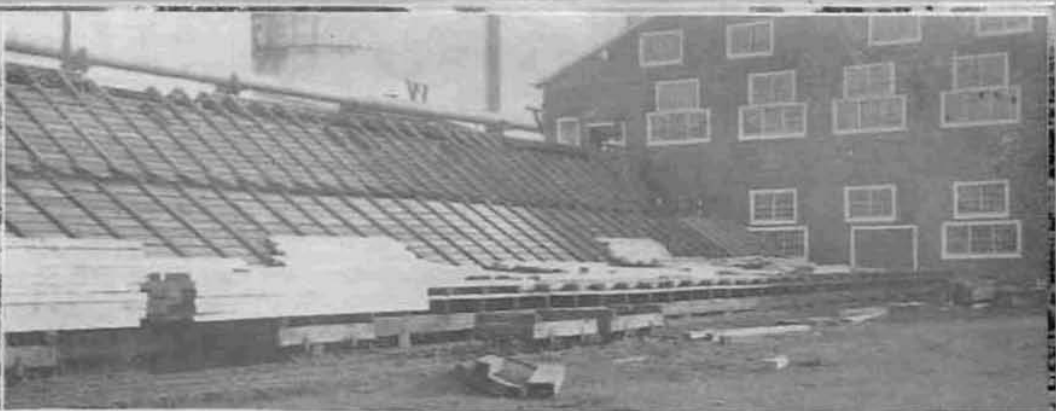
Above—Tie and Timber dock. Rails will be taken up from along this dock also. Loads will then be piled on bunks that will set on the ground, giving a downhill pull off the dock and making the work of stacking easier.
