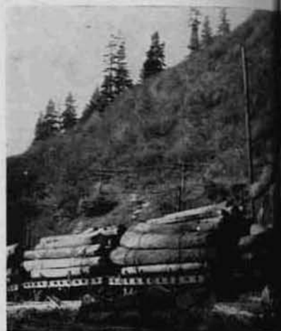
Avery landing . . . more than 16,000 poles and net of wire cable are to guard
