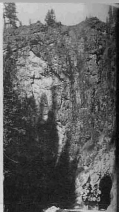
Tunnel on Camp 44 road up Fishhawk Creek. The region is extremely rough and offers a tough logging chance. Entire route of the eight mile road is flanked by steep cliffs.
