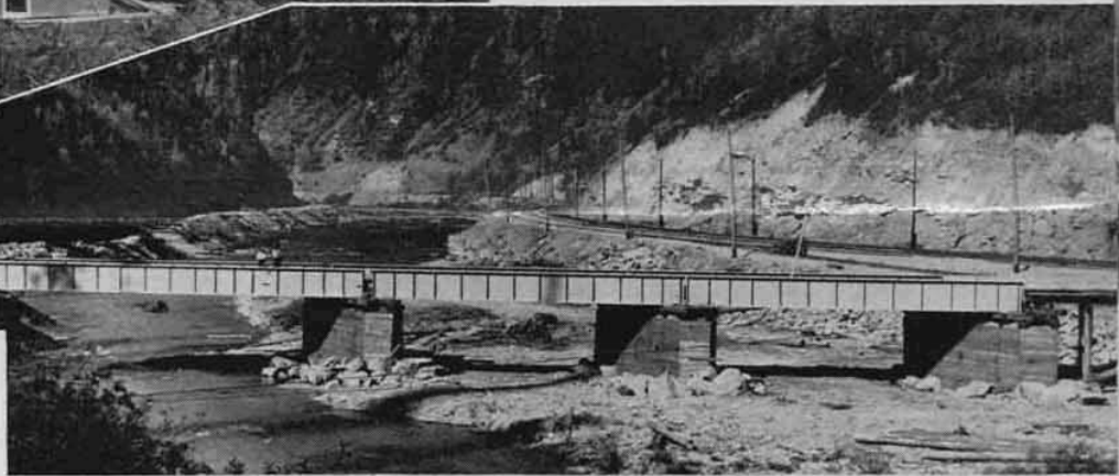
Bridge at Avery—steel girders from Coulee Dam—an entrance to landing.
