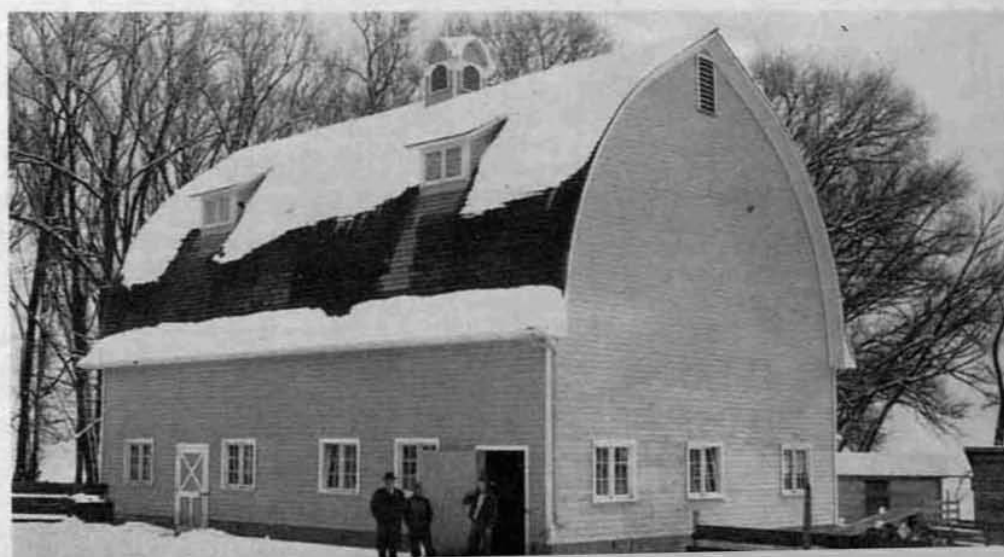
FRANK WOLF barn, Uniontown, Wash.—laminated arch rafters. In picture, lumber dealer PETE BUSCH, farmers CLIFFORD and LESTER WOLF.
