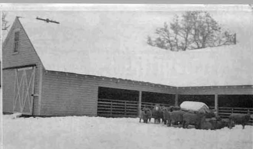
Poultry house at Frank A. Wolf farm, Uniontown . . . (Clifford Wolf in doorway) . . . designed by University of Idaho, Agricultural Dept. Has well insulated roof (eight inches of shavings), plenty of light, fine ventilation, houses a flock of 120 laying hens. Prize sheep, Washington State College.
