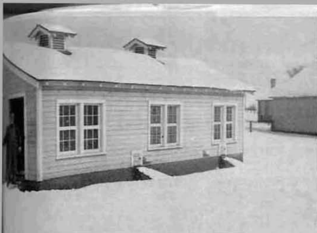
Poultry house at Frank A. Wolf farm, Uniontown . . . (Clifford Wolf in doorway) . . . designed by University of Idaho, Agricultural Dept. Has well insulated roof (eight inches of shavings), plenty of light, fine ventilation, houses a flock of 120 laying hens. Prize sheep, Washington State College.
