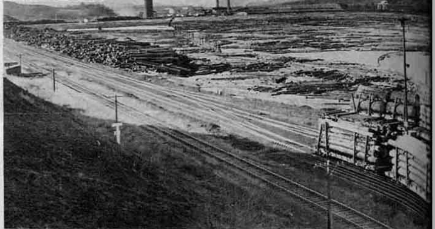
Upper left—Charlie Bailey, hoister, swings a big Ponderosa log aboard a log flat at the Stites landing. Note the flat car underneath the trestle that straddles the railroad track and supports the big swing boom loader. The car that is under the trestle in the picture will next be pulled into position for loading and the loaded cars pushed down the track toward the main line. Upper right—Six logs from the big tree at Camp 54 in late December make a carload. Total height of the tree was 186 feet 10 inches. It scaled close to 1,000 feet—an extremely large tree for Idaho White Pine. Above—Lewiston pond, 21 million feet more than last year, same date.
