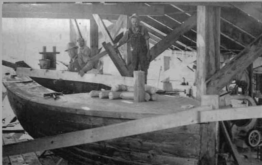
BOAT BUILDING UNDER CLEARWATER TIE DOCK —Boat Builder Fred Brautigam (on ladder) directs the building of a boat for the log pond at Lewiston. Under his supervision and with the help of Ralph Curtiss, center foreground, and Morriss McKown, background, the addition to the Clearwater Navy is fast assuming shape.
