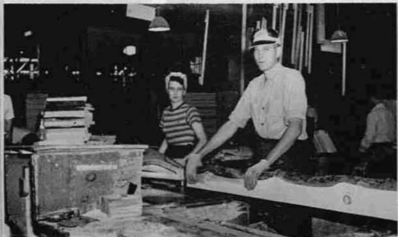
Below—Carl Twietmayer and Francis Roskawy. Twietmayer feeds lumber to the tumbler saw which operates from off an eccentric and comes up from under the table and inside the guard to cut the board into desired lengths. There are two such saws attached to each eccentric. Note the barky edge of the board, termed round edge by the trade. Roskawy stacks the cut-to-length pieces and passes them to ripper, Kenneth Dehnert.
