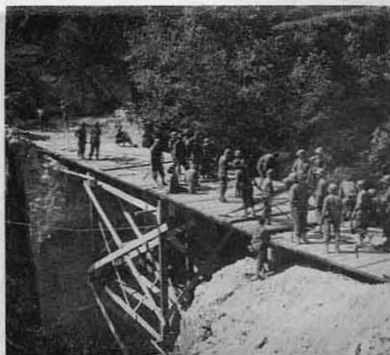
Above—TEN HOUR BRIDGE—It took Army Engineers ten hours to construct this bridge in Italy where lumber must accompany advancing troops to reconstruct bridges destroyed by the retreating enemy, else the route of troops and equipment is impassable or made miles longer.—Signal Corps photo.
