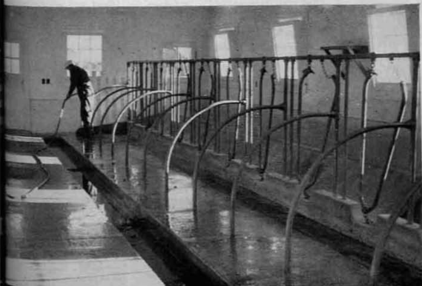
Below—The milking parlor was built with strict adherence to Health Department specifications. Water is at hand to quickly flush the concrete floor so that the milking parlor can be kept spotlessly clean.
