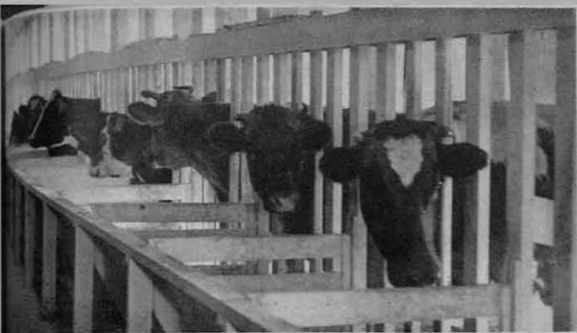
Above—Inside the barn that once was a stable for logging horses. Old stalls were torn down, the floor was ripped up and new stalls and mangers were built. Rebuilt windows, a drainage system, and a few coats of white paint transformed the old building into a desirable dairy barn.
