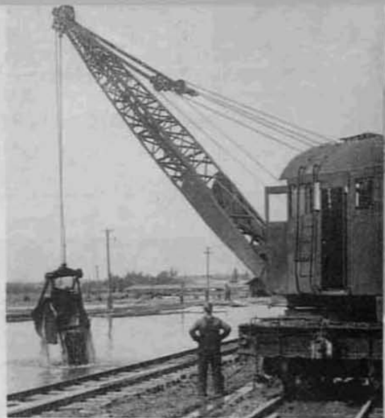
Dredging the pond at Potlatch . . . during the three week shutdown for repair of the sawmill the pond crew dredged the pond and slip area, also made necessary repairs to cat walks, booms, etc. The work was so arranged as not to interfere with dumping Camp 36 logs into the pond.
