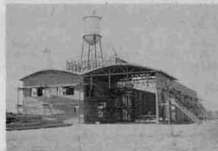
Building for Pres-to-logs plant at Sacramento in construction stage.
