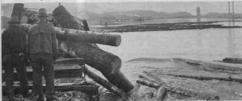
February 1945 averaged about 75 cars per day but August 1944 saw 2420 cars dumped into the pond. With backs to the camera are Casey Ellis and Charlie Moore, two of the unloading crew. Note dangling links of the releasing stake pocket. Upper right—long train of loaded log flats passing by the big deck of logs (safety measure against winter shutdowns).
