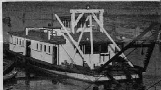
Above—The dredge Clara. Hers is a steady job despite the fact that the Clearwater deserves its name during most of the year. Silt accumulates at a fast pace, must be sucked up and discharged out of the pond.
