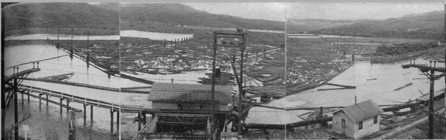
Above—The Clearwater pond—310 acres in size but with a total backwater of 760 acres. Center picture shows shelter over log slip and washer. In the foreground of picture at right top is pond shack where extra clothing is kept just in case of an involuntary bath. At right picture is deck of logs along hot pond unloading dock.
