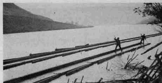
Above—The long fin booms are periodically hauled out for inspection and repair then put back into the river. It's no easy task.
