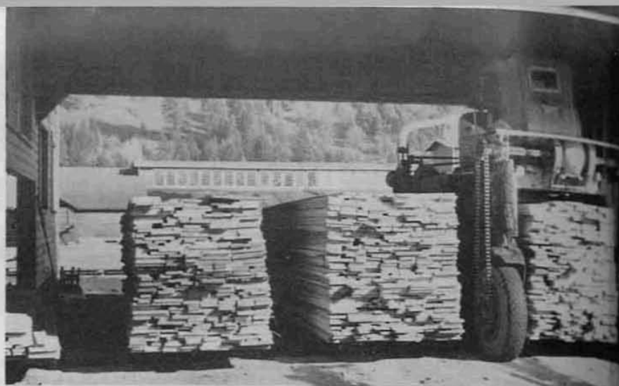
The straddle bug at Rutledge places another load of lumber on the conveyor chain that will carry it into the stacker building, a part of the new dry kiln set-up at Rutledge. Although lumber inventories at the three mills are now lower than ever before in the history of the company (and Rutledge lower in proportion to its shipments than either of the other two mills), 107 cars of lumber left this plant in February 1945 as compared to 77 in February 1944.
