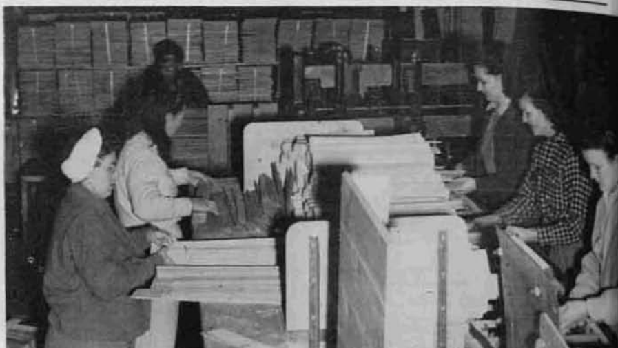
Above—The machine for assembling slats and cleats preparatory to stitching them into veneer shook covers is one of considerable complexity. Girls arrange the slats on a traveling chain that carries them to the stitcher.
