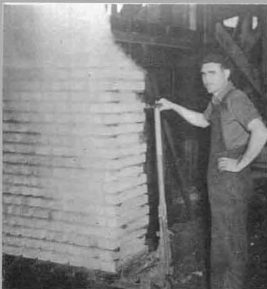
Above—Orville Luster pulls a load of steaming blocks from the steam box. Steaming time varies from 2½ to 5 hours depending on thickness of blocks.
