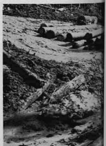
Below—the landings were muddy places of the skidding pan. Logs soon became partially covering them to a depth of several inches.
