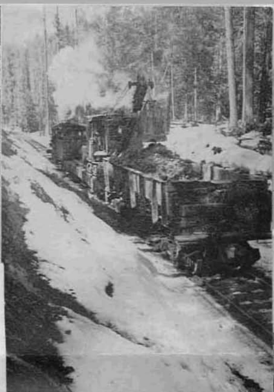
Above—The ditching crew at work cleaning out the cut between Camps 55 and 59.
