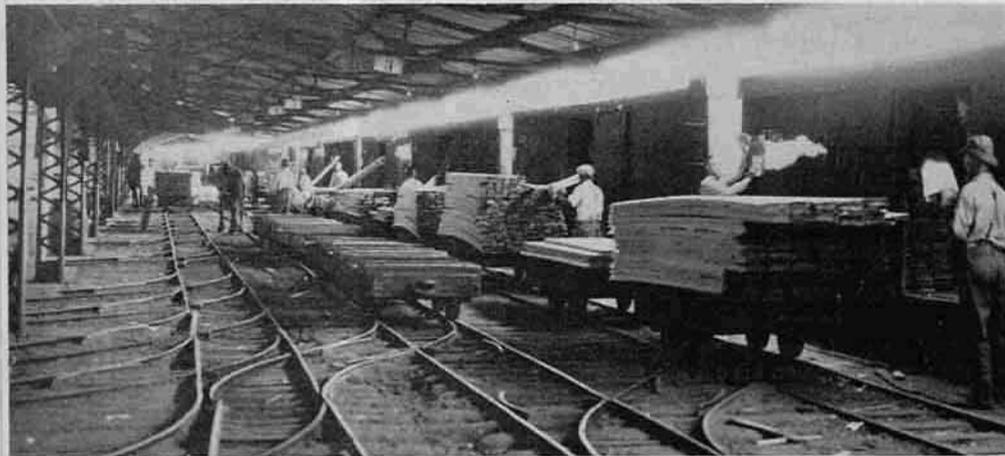
Above—Finished lumber once moved from planing mill to loading dock over these rails, towed by horses.
