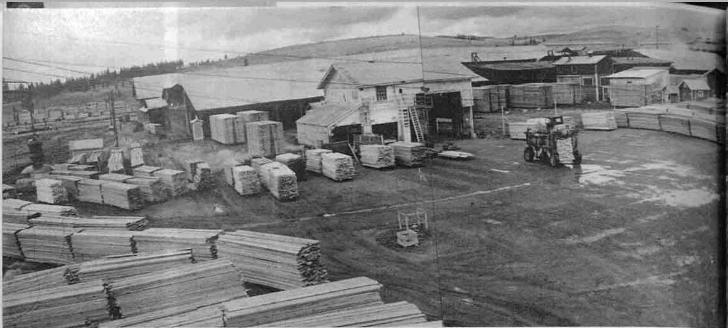
Above—Panorama of Potlatch green chain, stackers and yard between. The paving eliminated weeds, fire hazards, dust. Low spots have yet to be graded out to assure proper drainage. When clear of lumber piles the paved area between green chain and stackers is long enough to permit Piper Cub to land and take off.
