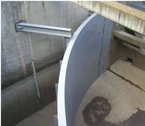
Figure 1. A) Narrowing of the junction pool wall and B) aluminum/steel plating on lower eleven weirs in the fish ladder at Lower Granite Dam during 2006.
