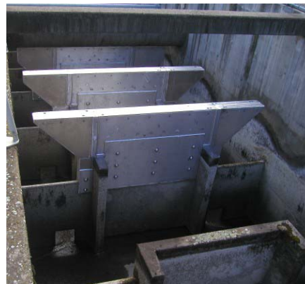
Figure 1. A) Narrowing of the junction pool wall and B) aluminum/steel plating on lower eleven weirs in the fish ladder at Lower Granite Dam during 2006.
