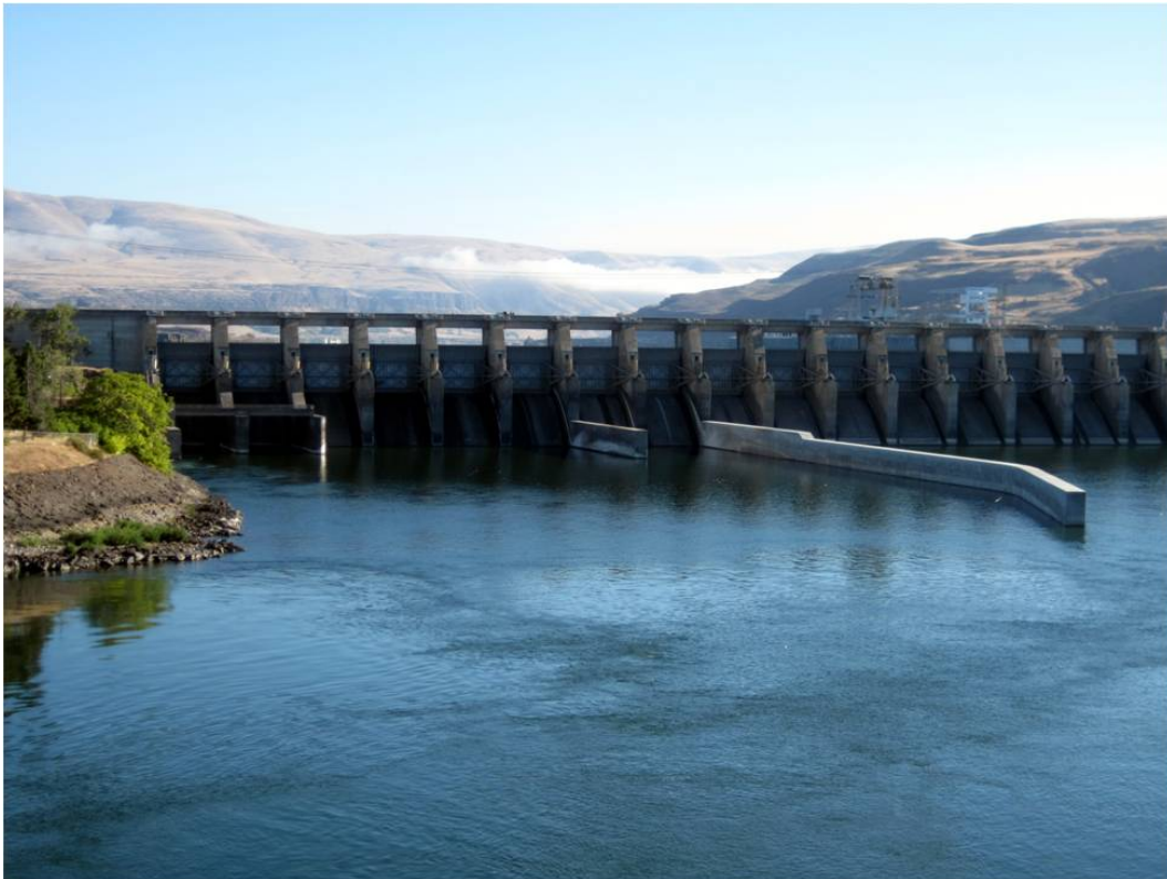
Figure 1. Photograph of spill walls at bays 6/7 (left) and 8/9 (right) at The Dalles Dam in 2010.
