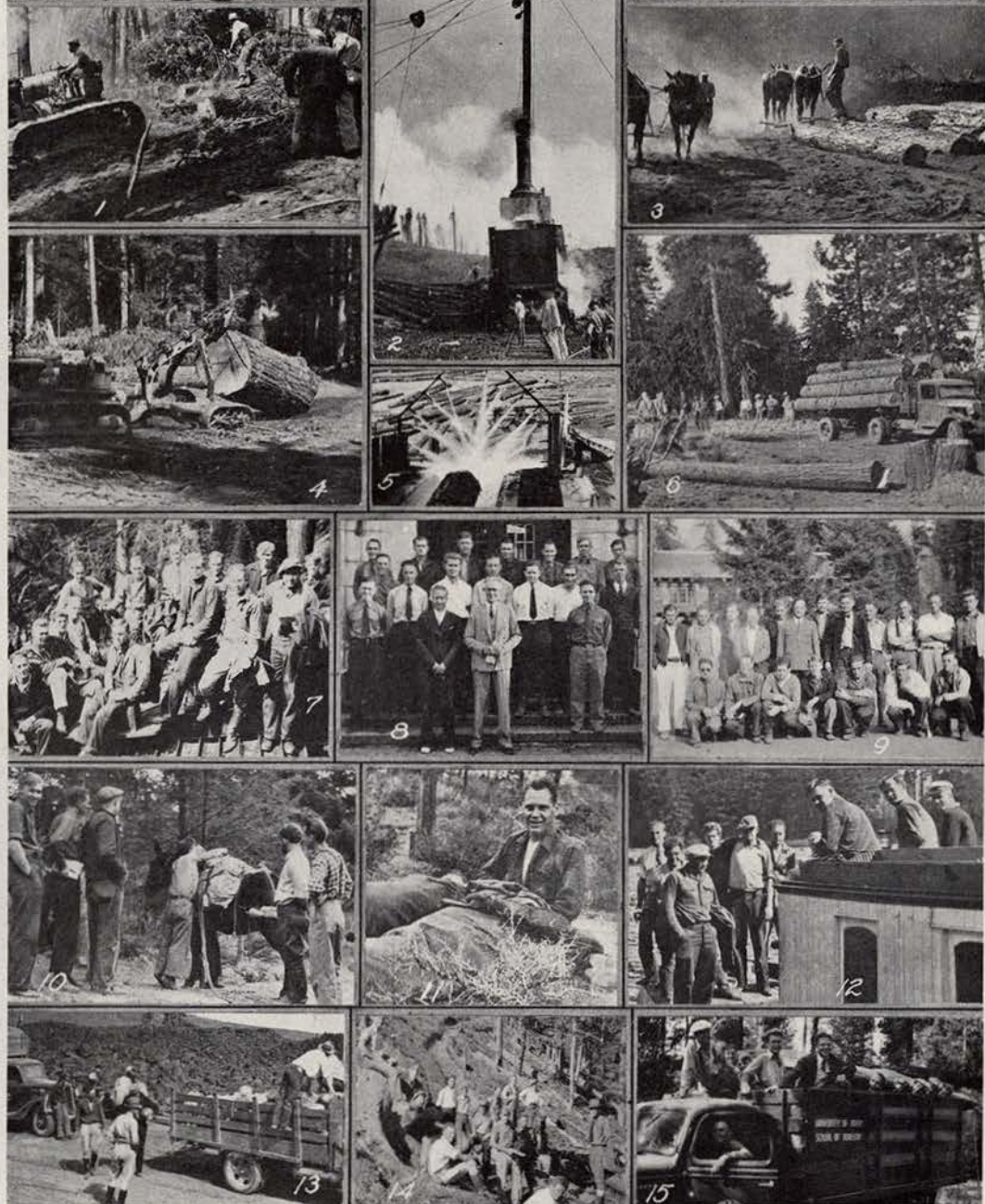
1. Tractor logging in Ponderosa pine near Ellensburg, Wash. 2. Logging with a "skidder" near Seaside, Oregon. 3. Team logging in Ponderosa pine near Bend, Ore. 4. Vencer logging with a "Cat" and a Fairlead Arch near Morton, Wash. 5. The log's last stand. It is a short step from here until it is cut into lumber. 6. Truck-haul near Bend, Ore. 7. Taking a "five". Can you find Ted Pierson? 8. Seniors looking their best with Dean D. S. Jeffers, center, and Leslie Larson, center left. 9. Seniors posing with Major O. A. Tomlinson, center in uniform; Prof. Alexander, center left; and Prof. A. M. Sowder, center right. 10. Team mates "Goliath McKeever" and a government mule demonstrating the diamond hitch. 11. "Mourning" in the morning. Eh Paul?? 12. Seniors afloat on Silcoos Lake. 13. A. M. Sowder supervising a "mellon snitch" on McKenzie pass near Bend, Ore. 14. Ken, Davis and C. James showing the boys a broadcast burn in Hemlock on the Deception Creek Experimental Forest, Coeur d'Alene, Idaho. 15. Lowering the top for a low "bridge" while enroute.
