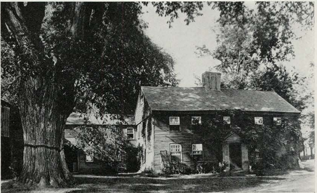
The Abbot house, built in 1685 at Andover, Massachusetts, of white pine. It is still standing and sheltering mankind.
