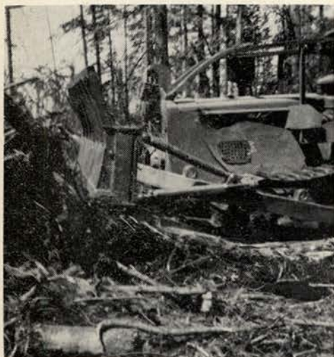
Bulldozer Piling Up Slash
