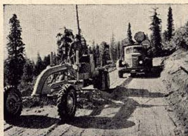
Motor graders for building and maintaining truck haul roads, maintaining fire lanes, leveling camp sites.
