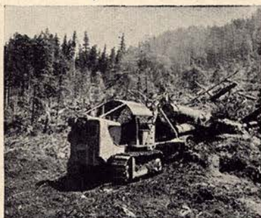
Tractors for yarding and skidding logs, building roads, clearing landings, cutting fire lanes.
