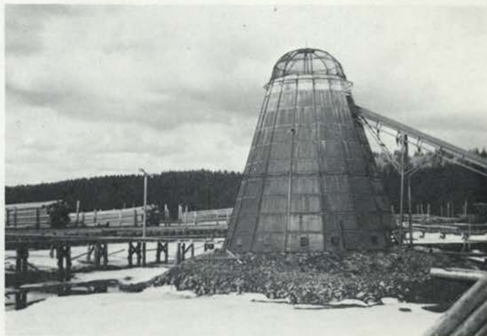
Red Cedar pole yard in Northern Idaho. This Burner is no longer used to burn Cedar bark. (Photo by Scrivner)
