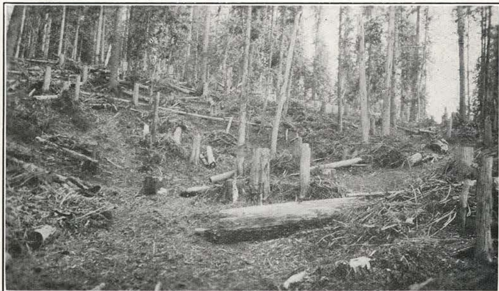
Brush piled ready for burning.
