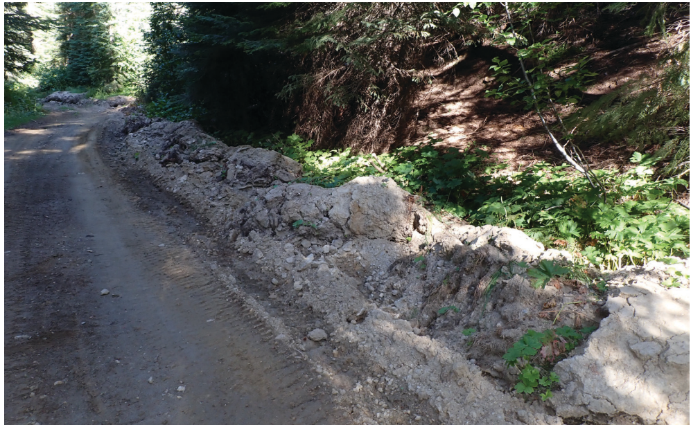
Picture of a berm of dirt (above) moved to the side of FSR 1826, suggesting, with tracks, the presence of heavy machinery on this road prior to any project authorization.
