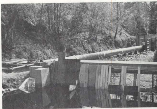
Fig. 14. Downstream view of the 30.5 m culvert facility showing the position of the headbox, tailbox and dam (1974 and 1975).
