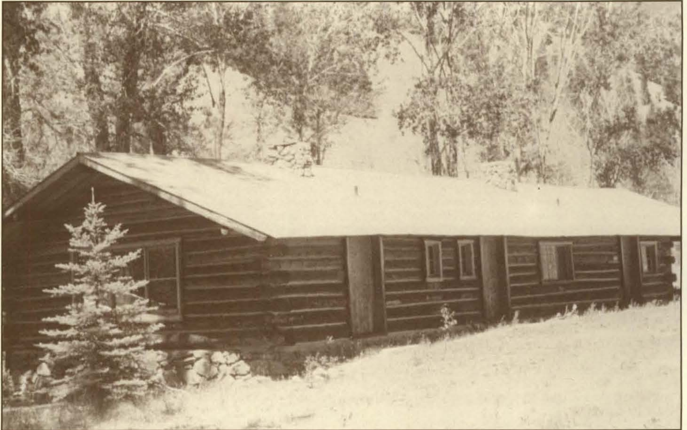
The Lanham cabin was disassembled, transported to the Cabin Creek airstrip, and airlifted by Idaho National Guard helicopter to Taylor Ranch, where it was reconstructed.
