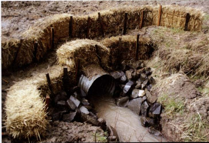
Properly installed and protected culvert.
