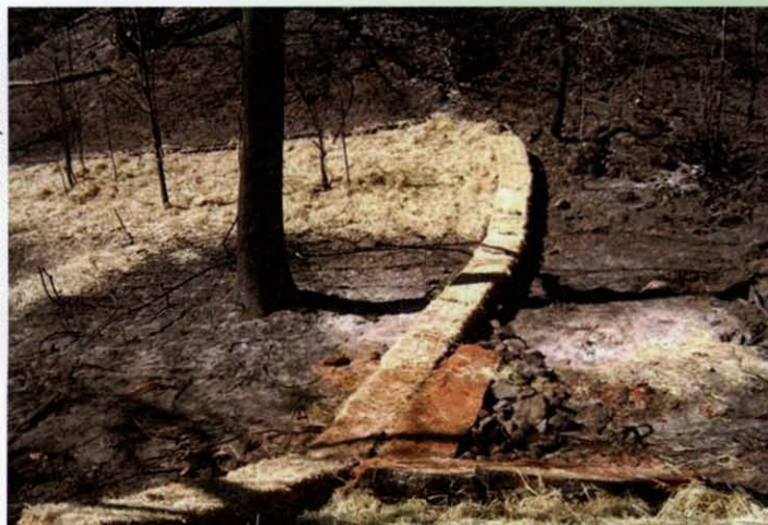
Straw bale check dam.
