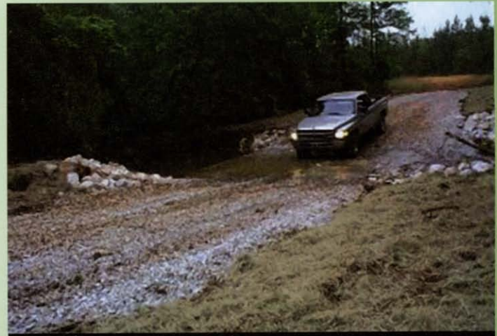
Armored stream crossing.
