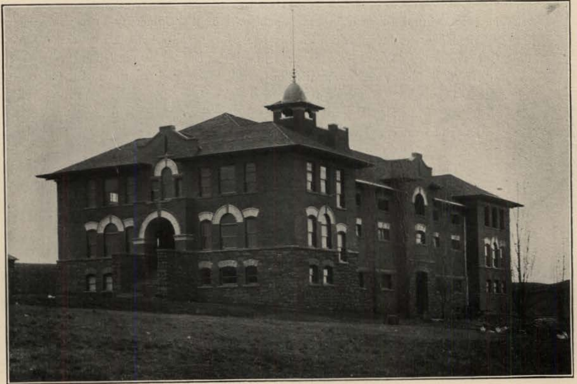
ARMORY AND GYMNASIUM
