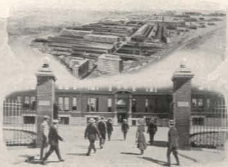
MAIN PLANT GENERAL ELECTRIC COMPANY
