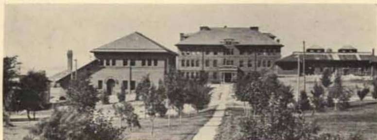
VIEW NORTH FROM ADMINISTRATION BUILDING
