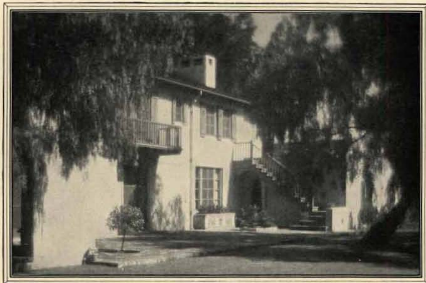
HOME FOR C. F. PAXTON, PASADENA, CALIFORNIA. REGINALD D. JOHNSON, ARCHITECT. CRANE SANITARY EQUIPMENT INSTALLED BY THE SOUTH PASADENA PLUMBING COMPANY
